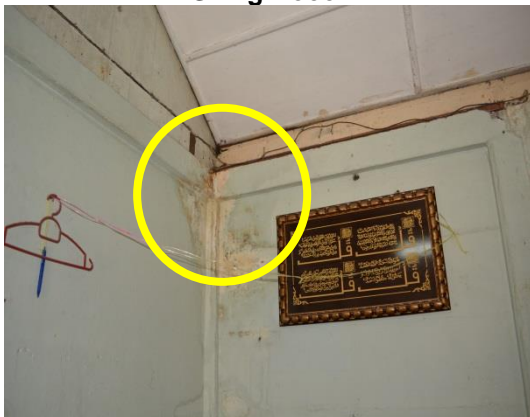
Gambar 3.5 Siling Bocor
